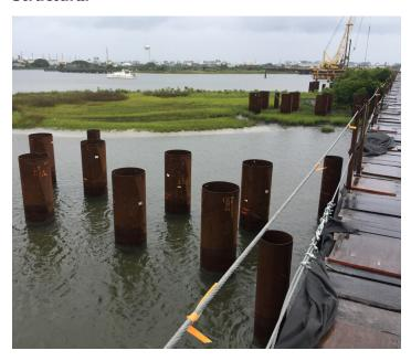
Spiral welding, the process used by AMERICAN to manufacture AWWA pipe cylinders, can also be used to manufacture steel cylinders for structural applications such as:
