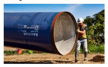
The conservative wall thickness recommended for the handling of steel pipe during the manufacturing, shipping and installation phases of a project is dependent on the type of coating and lining specified by the owner or owner's engineer. Steel pipe with flexible coatings and linings (e.g., polyurethanes, epoxies) should have a minimum diameter/wall thickness ratio (D/t) of 288. For conventional cement-mortar-lined steel water pipe, the recommended D/t ratio is no more than 240.
