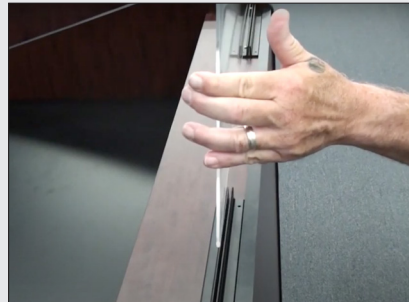
Step 2 - Fit Safety Shield into rail(s)
