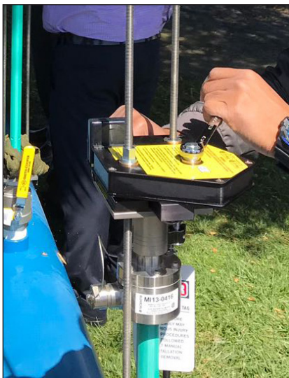
Figure 23. Inserting the sensor with the insertion tool
