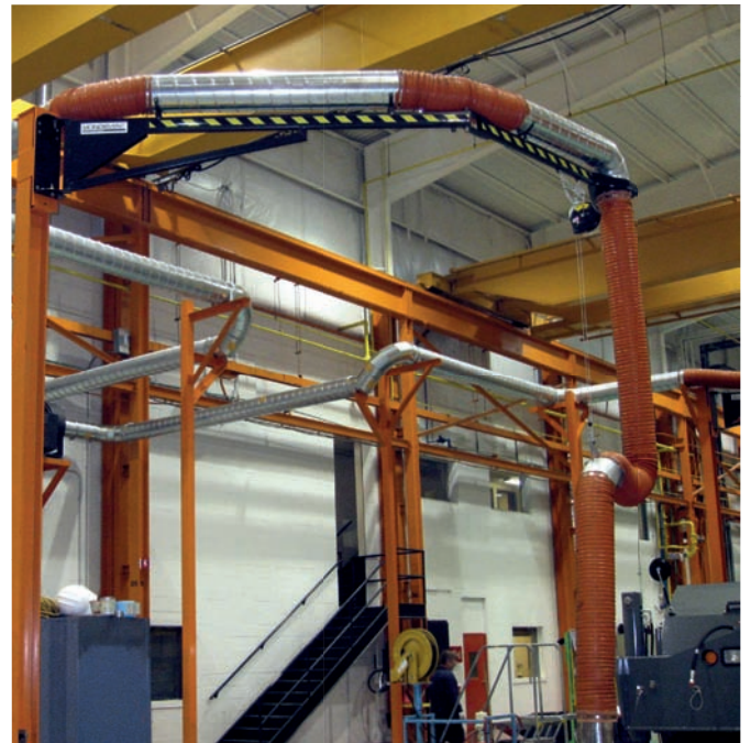
11000 Series Overhead PAC (Pivoting Articulated Crane) System, with 4000 Series Hose
