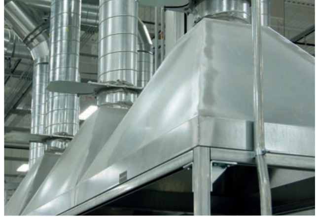
Overhead Canopy hoods for high temperature application, shown with optional blast gates
