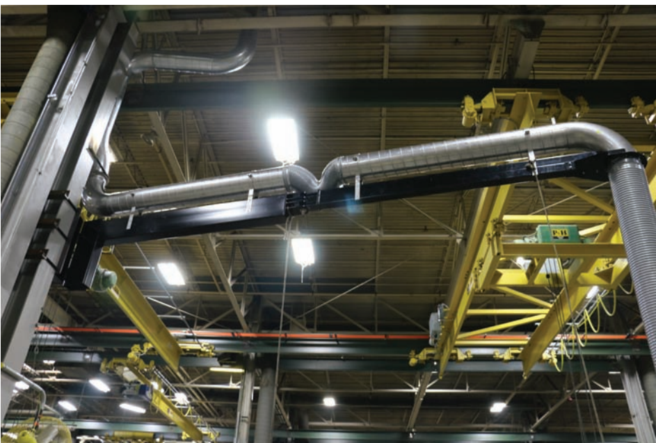
Heavy Duty PAC, 24', High Temperature Hose Drop
