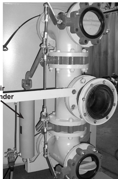
Series TFB pneumatic actuation system in filter position
